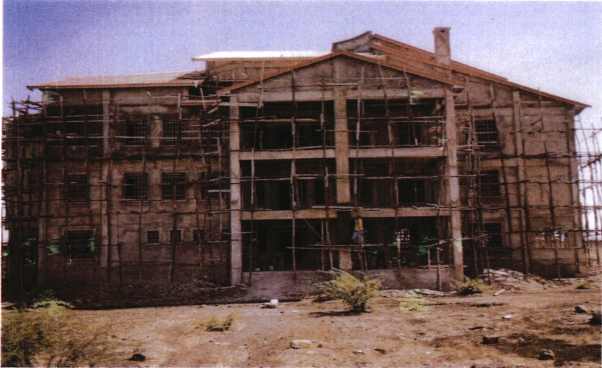
Photo 8: CWSK Integrated child and family centre - Isiolo –house block unit 1
