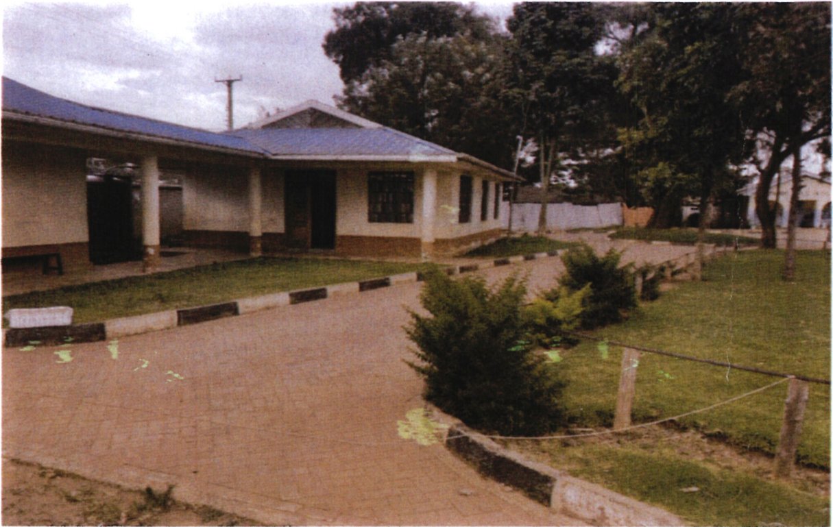
Photo 10: CWSK Nanyuki – Integrated child and family centre – Health centre, guard house, parking complete
