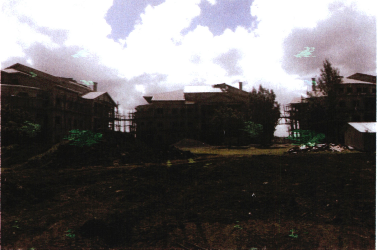
Photo 11: CWSK Nanyuki – Integrated child and family centre – Three house blocks above
