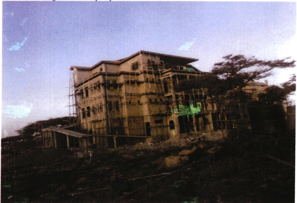
Photo 9: CWSK Integrated child and family centre - Isiolo –house block unit 2
