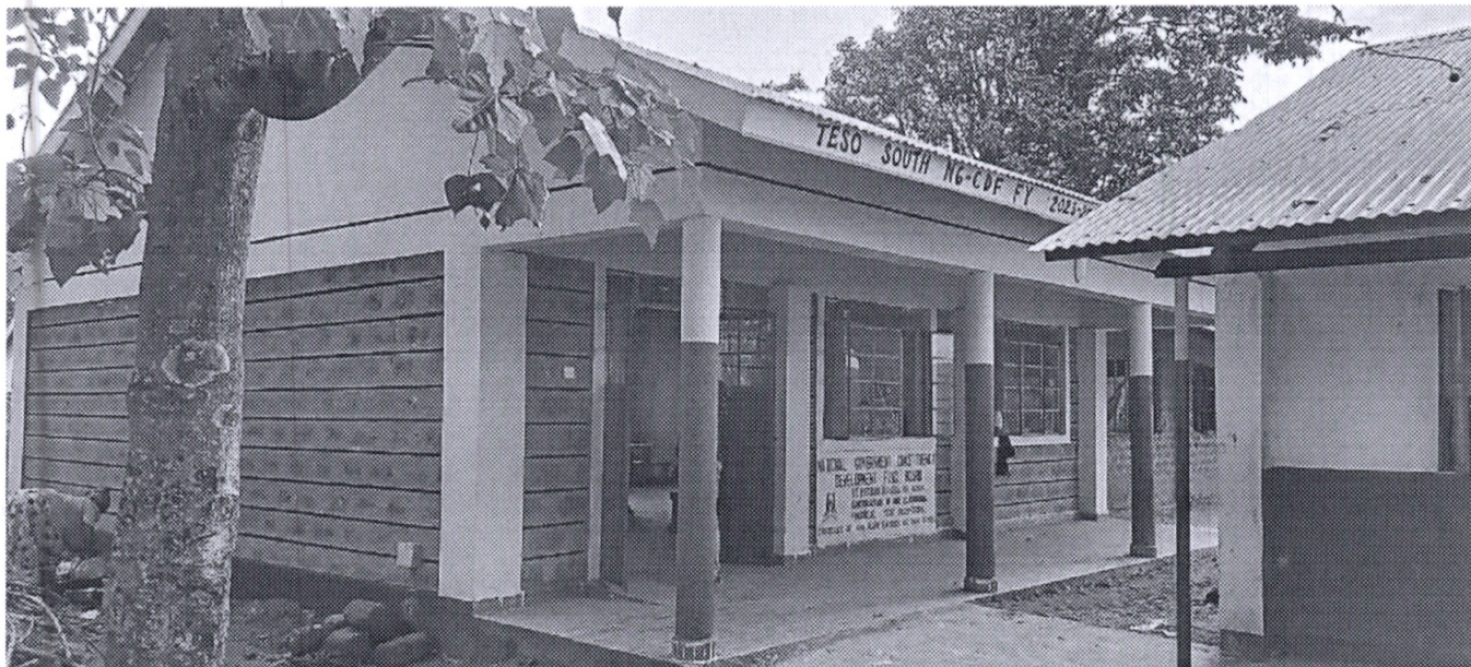
Figure 3: Kosera Primary School– Construction of one classroom
