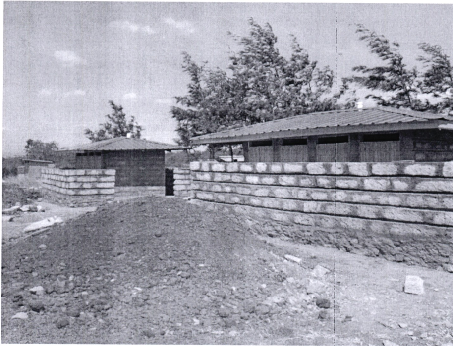
FIG 1.1 Kanthungu Primary School toilets under construction
