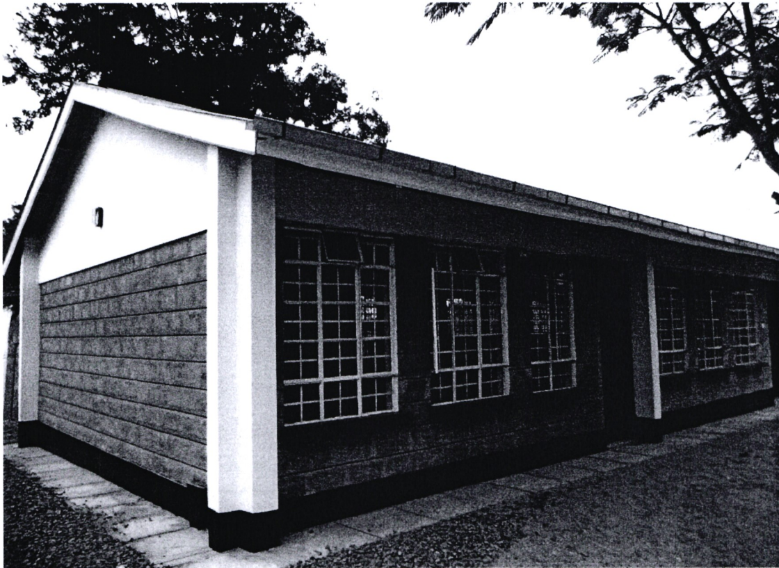
Newly constructed CDF offices at Makueni County
