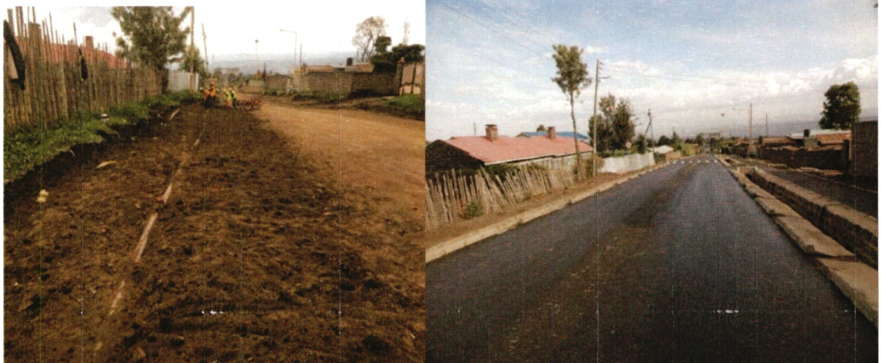
Figure 1: Before and Completed section of Kirinyaga Roads in Kirinyaga County
