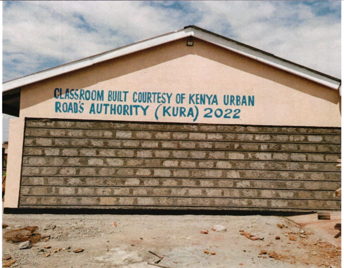
Figure 8 : Completed Classroom of Lake Baringo Secondary School.
