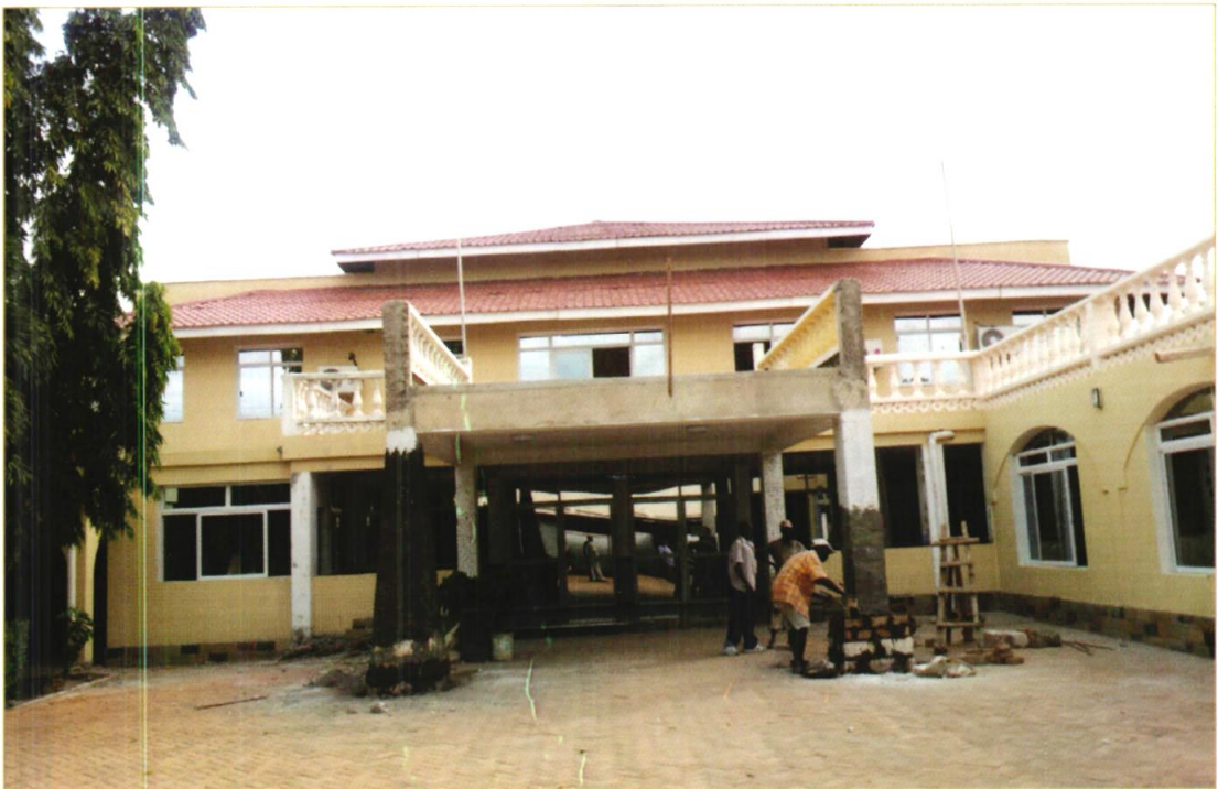
Kilifi Assembly Chambers under construction.
