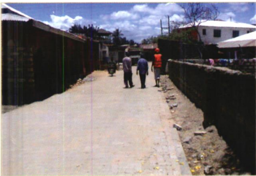
Watamu Township Cabro works.
