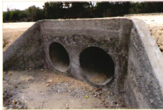
Marafa Chamari Road (culvert installation)
