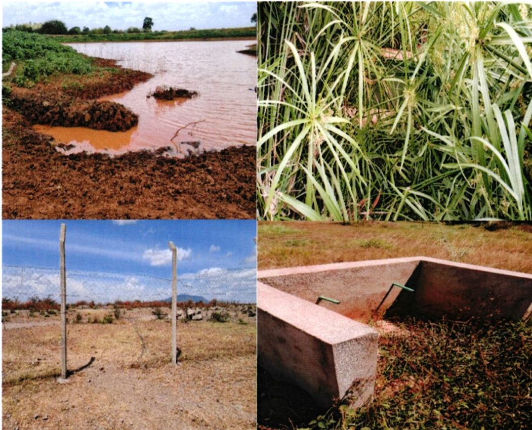
Figure 13: Photos showing lack of maintenance in dams and pans without custodianship
