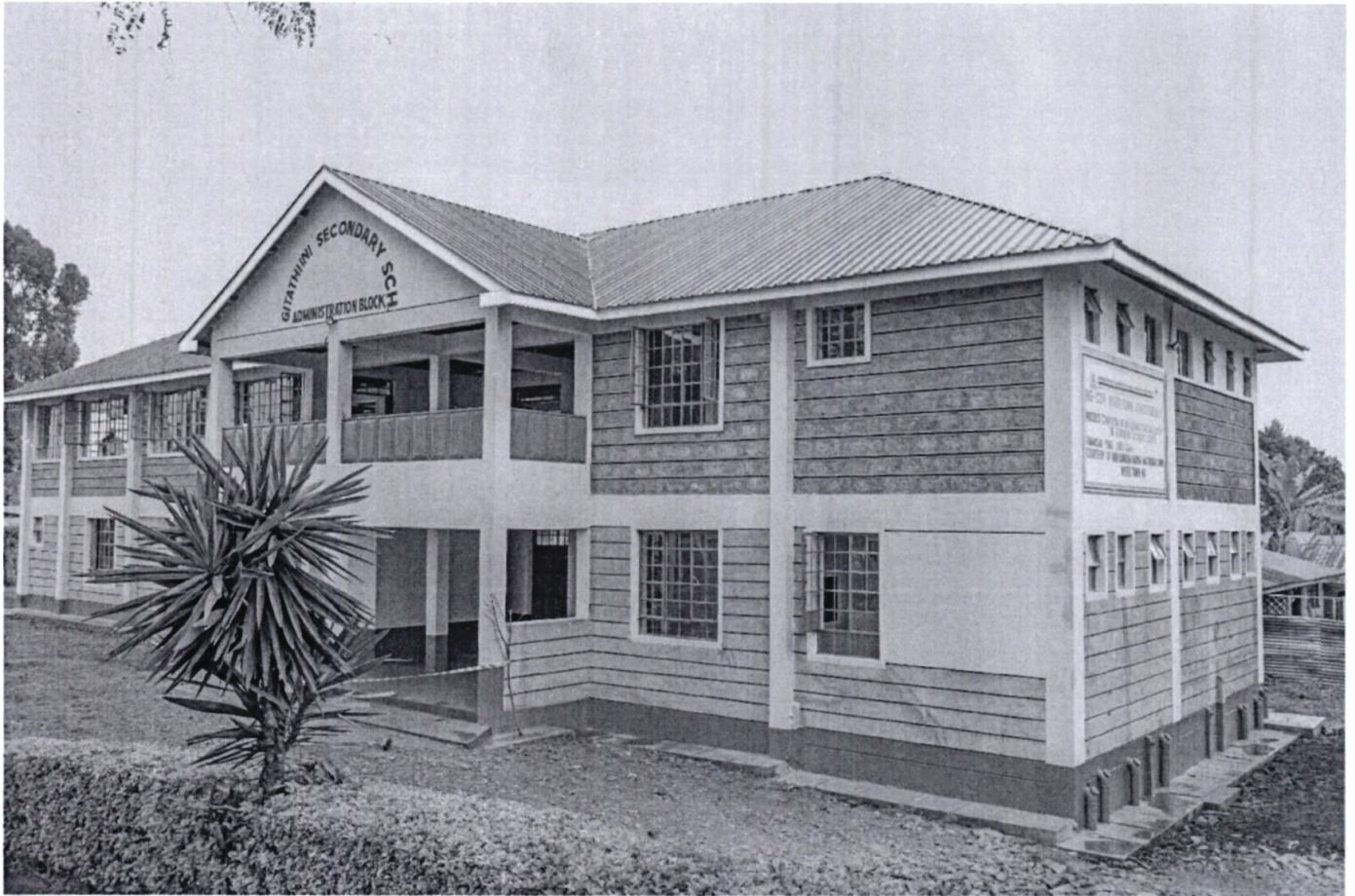
New Constructed Administration Block at Gitathi-ini Secondary School
