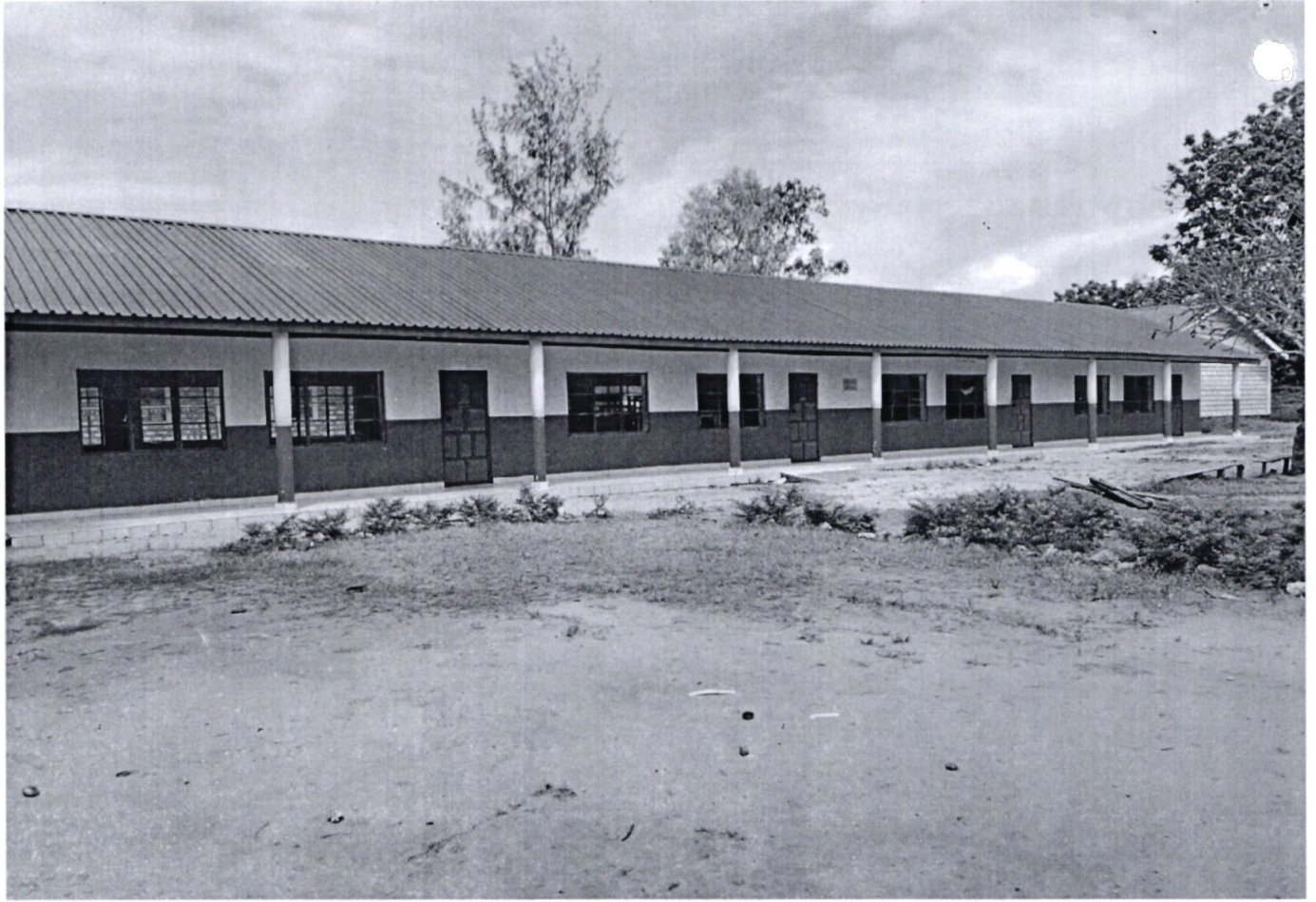
Galu Primary School Renovation of 4No. Classrooms.
