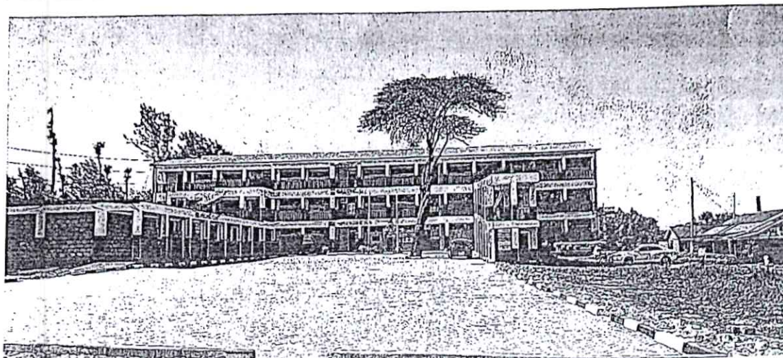
Cabro project at Vet Lab Sec School
