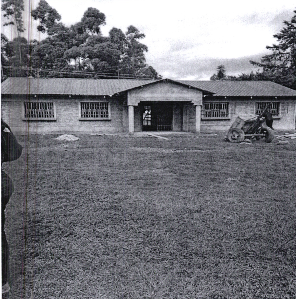
On-going chesunet primary administration block
