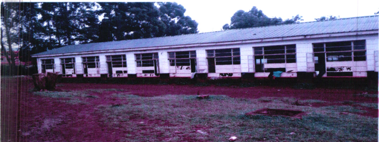
Sosiani primary school replacement of asbestos roof with iron sheets
