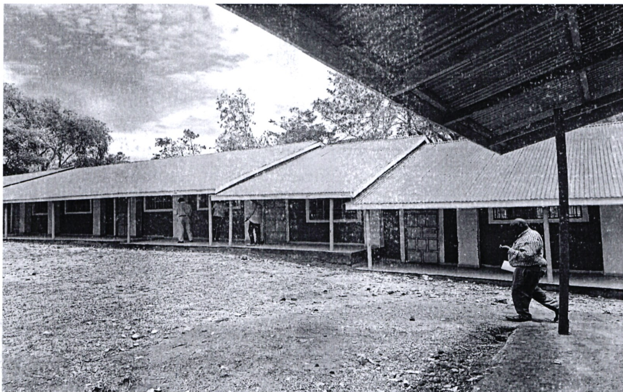
Sota Primary School, Construction of 4 No. classrooms
