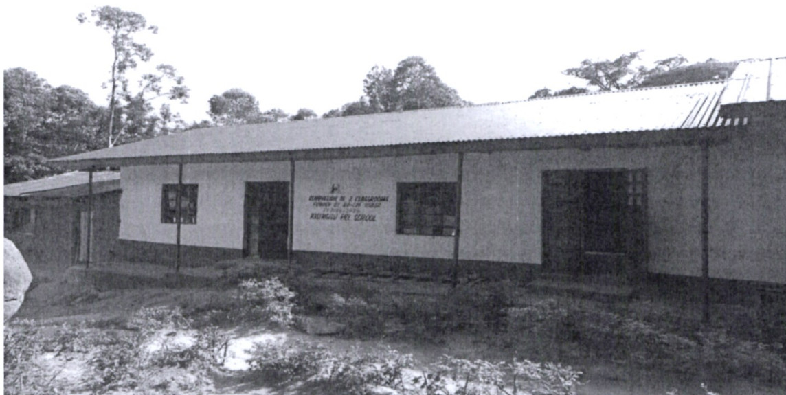
Figure 2: Kisingilu Primary School – Renovation of Two Classrooms
