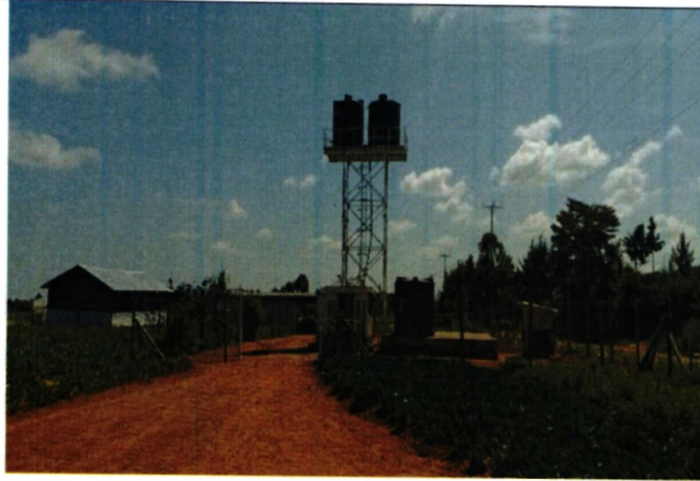
Borehole, water harvesting & storage in Laikipia
