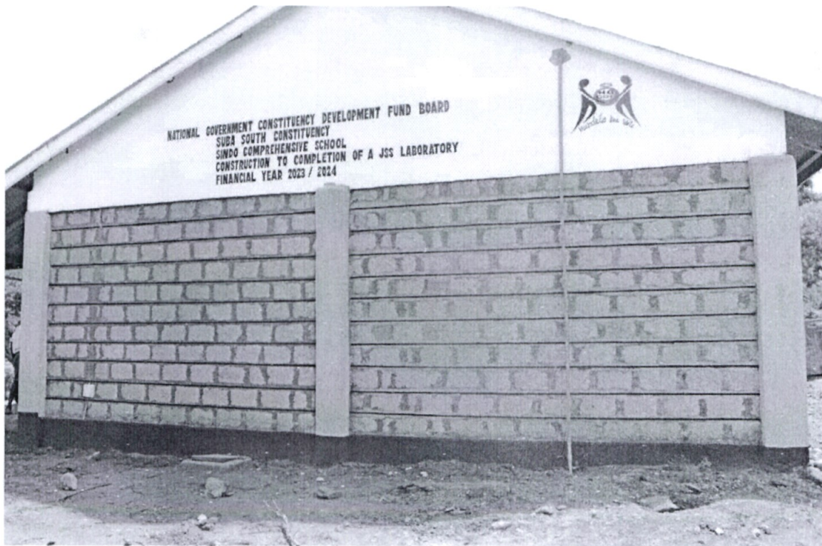
Fig 2: JSS laboratory at SIndo Primary School
