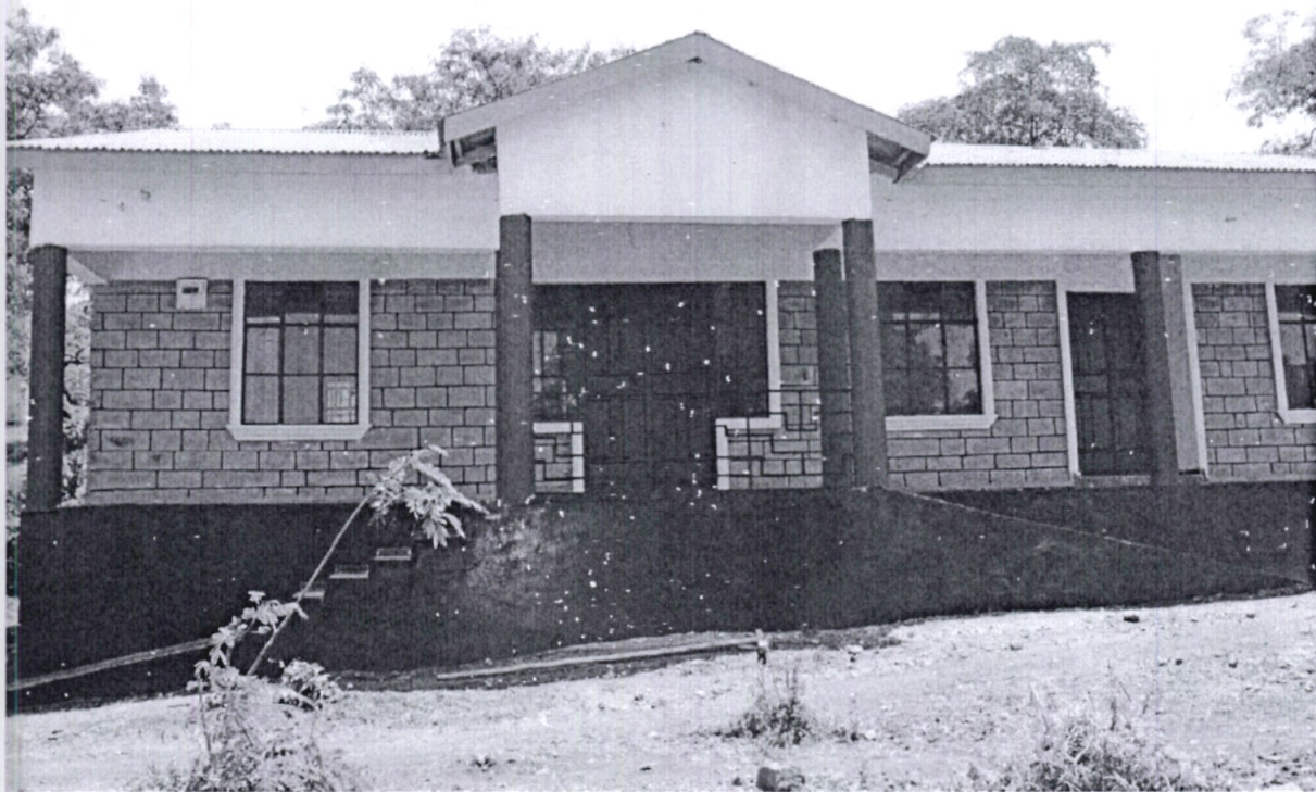
Fig 1: Administration Block at Osiri Primary School
