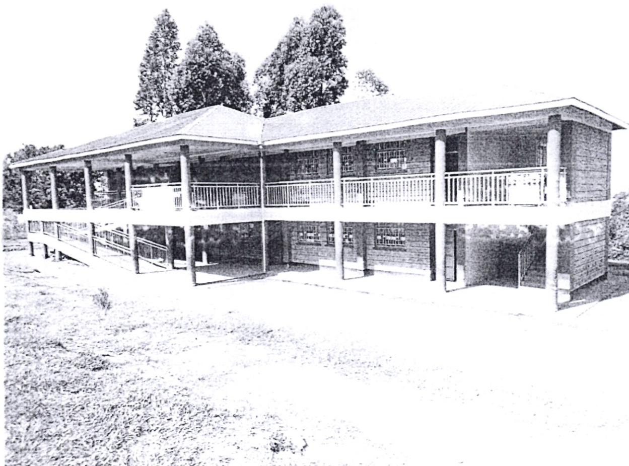
The complete 6 classroom block at Sikimbilo Primary School
