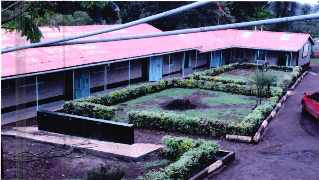
Renovation of 12 classrooms at Njenga Karume Primary School.
