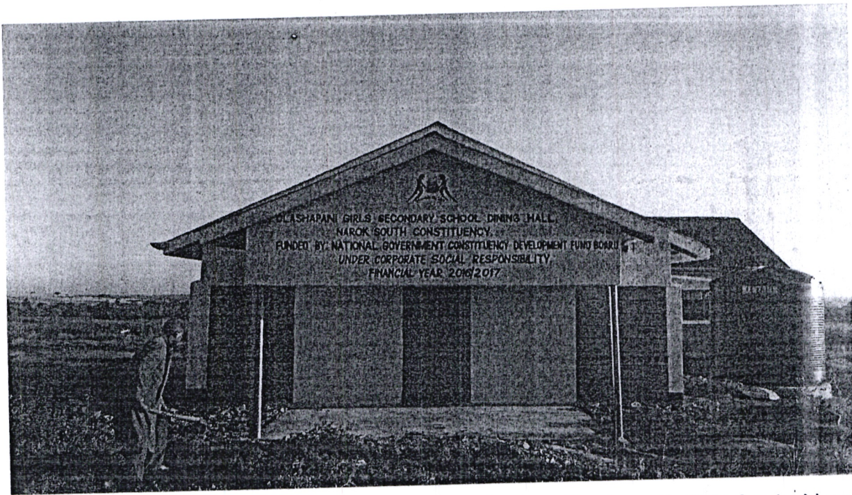
Installed water harvesting facilities on a dining hall at Olashapani Girls Sec in Narok South Constituency
