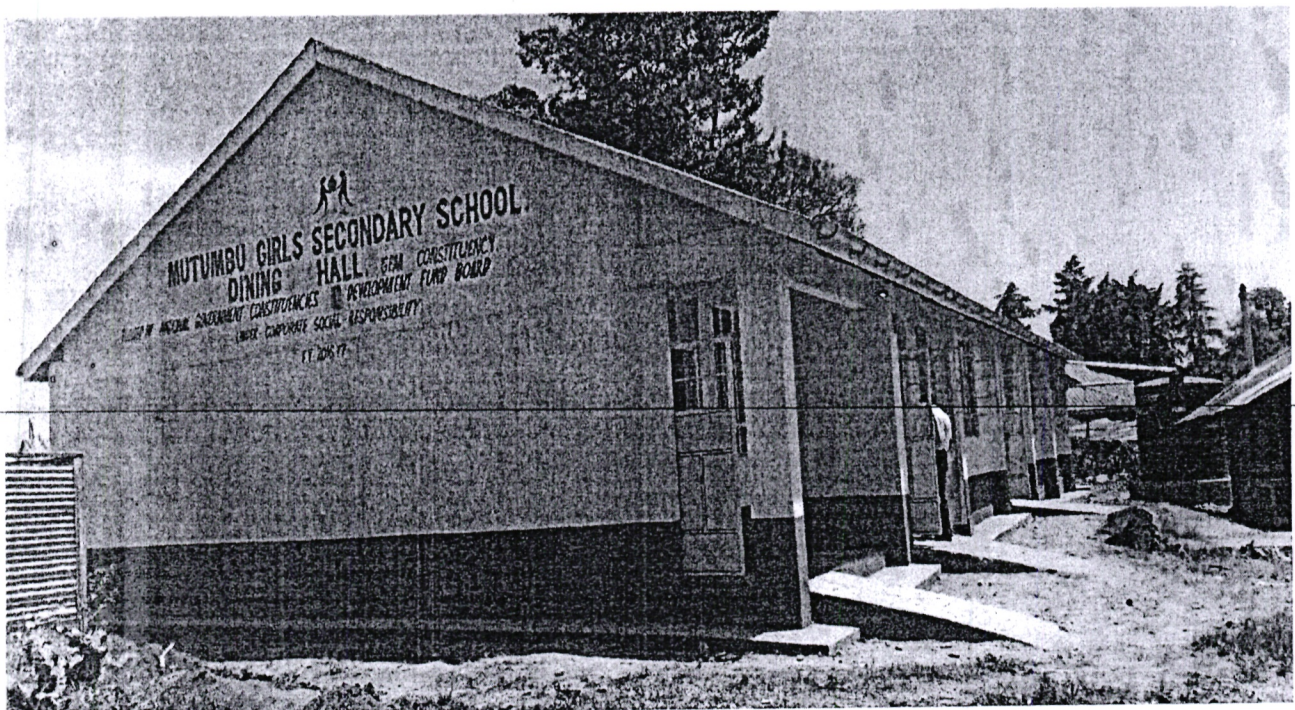
Installed water harvesting gutters on a dining hall at Mutumbu Girls secondary school in Gem constituency (completed in 2019/2020 fy)
