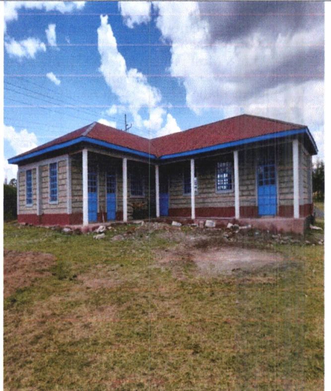
AIC Ndulele Secondary ; construction of Laboratory.
