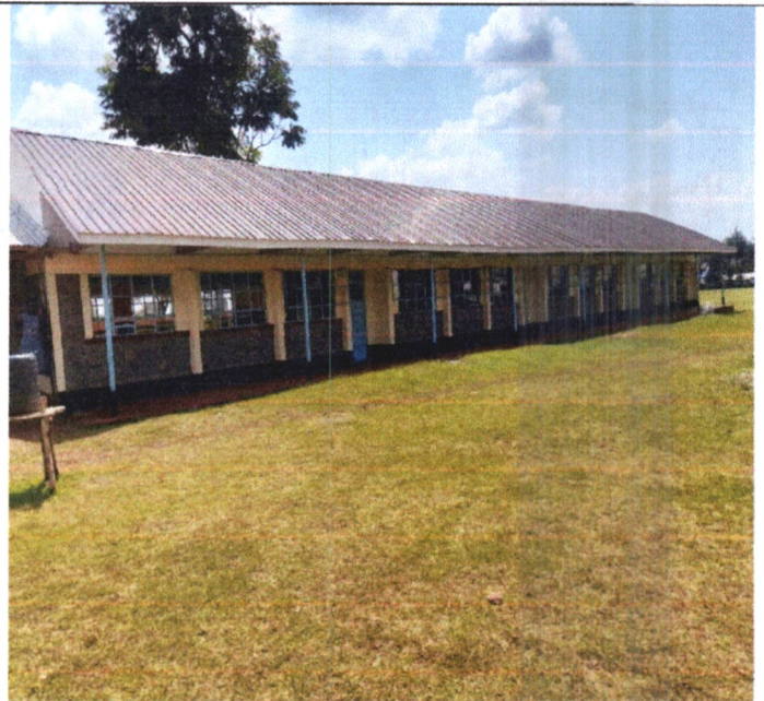
AIC Kaigat Primary School: Construction of Four classrooms
