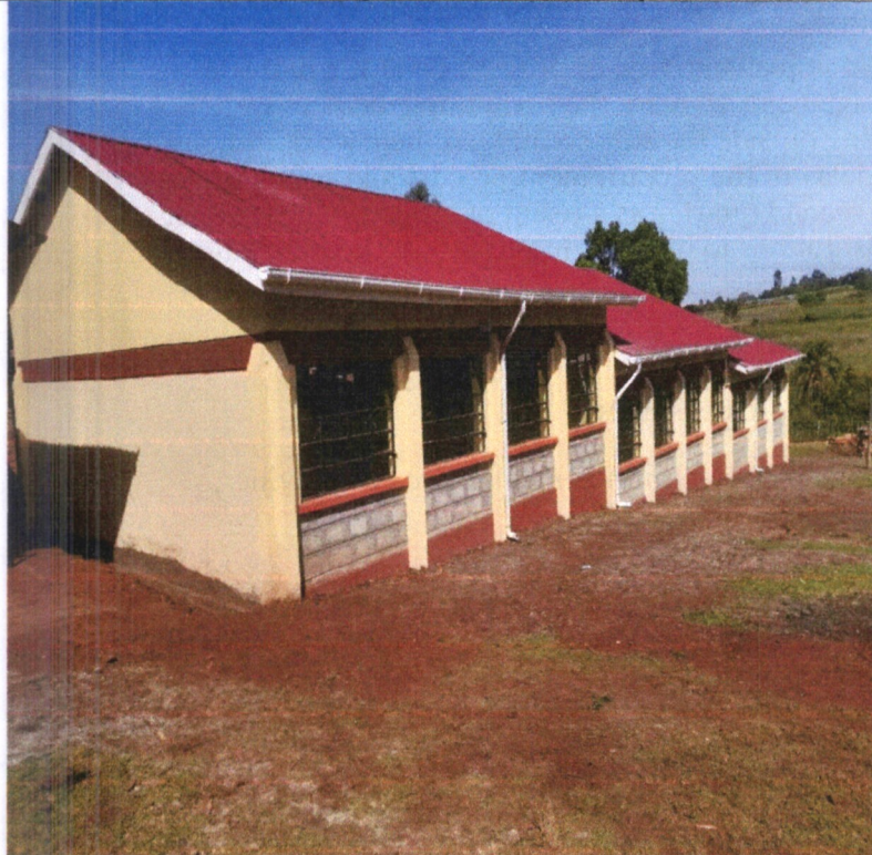
Kipkaren Township Primary School: construction of Four classrooms.
