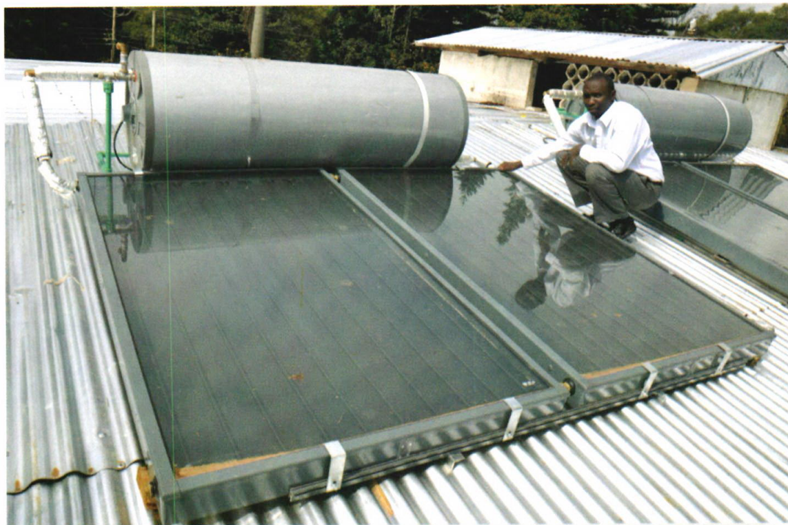
Inspecting a solar water heating installation.
