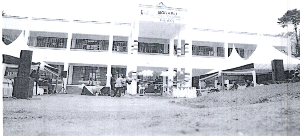
Construction of Borabu NG-CDF office with ground and 1 st floor hall and offices at Kshs 42,000,000
