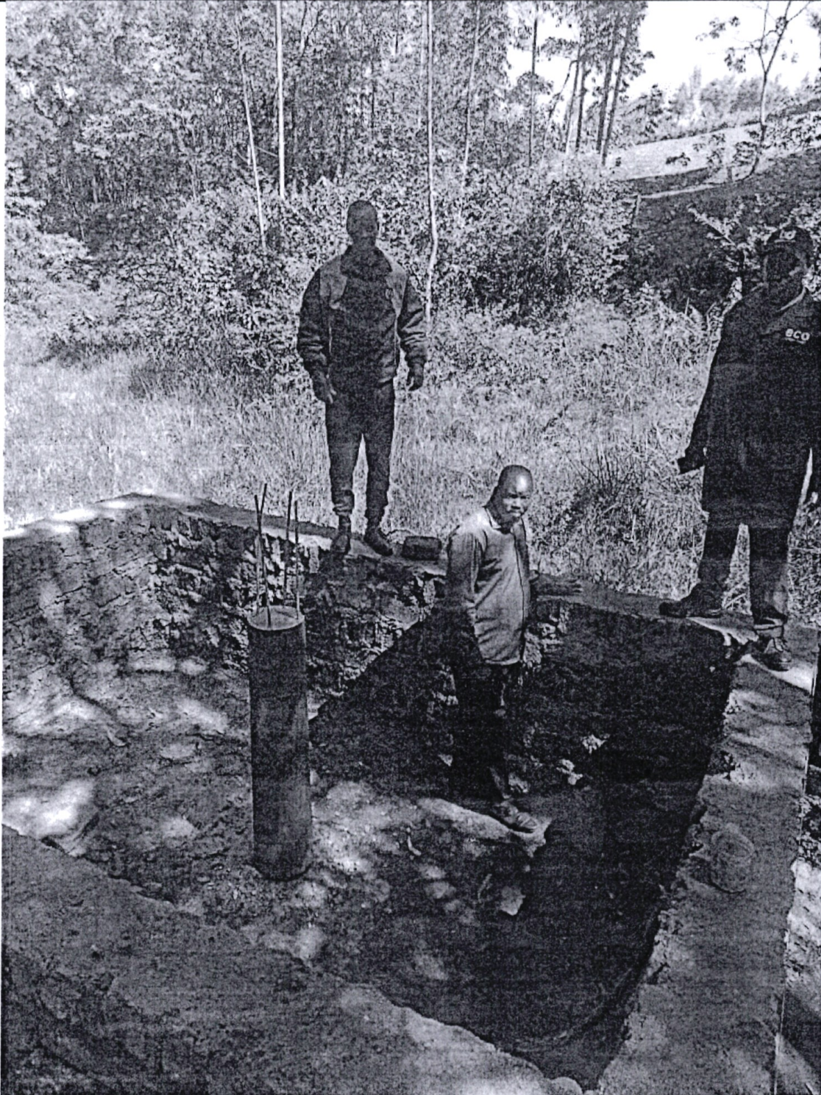
Kombe water project (Water Tank Foundation).
