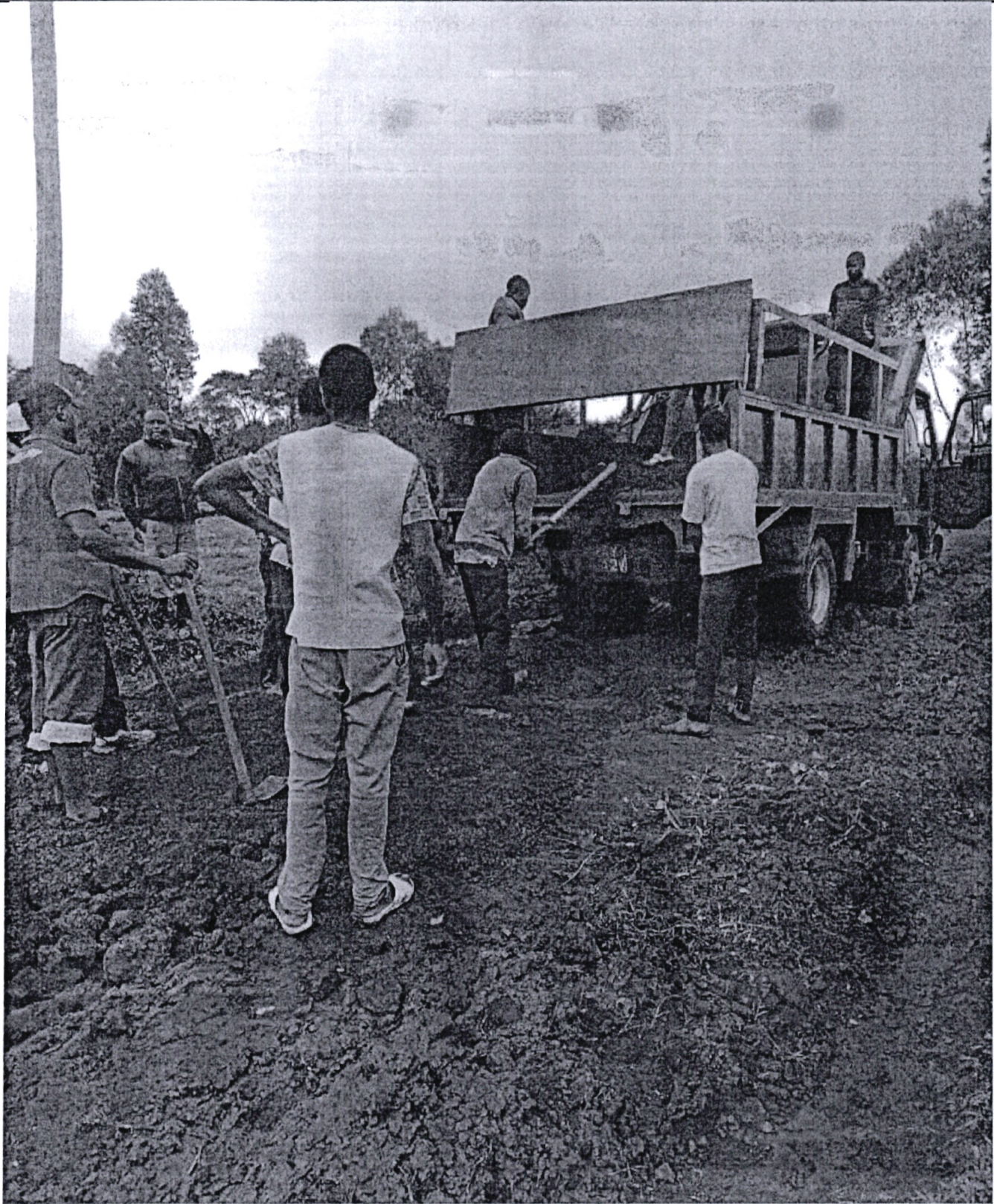
Road repair works in Kipchabo Catchment Nandi County.
