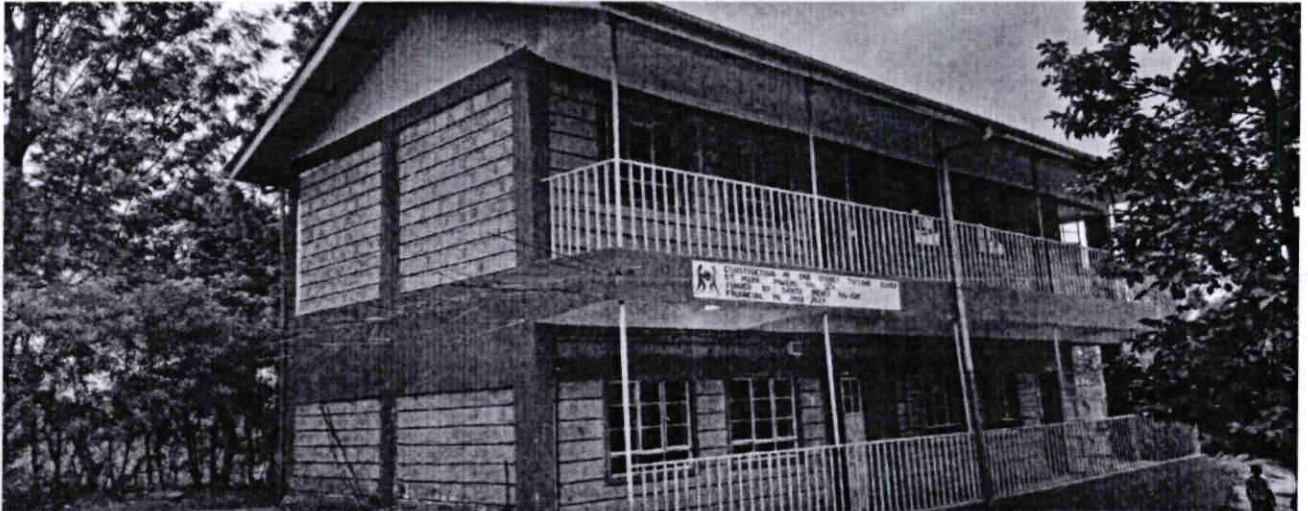
Photo of St Marks Mweru Primary School Classrooms in South Imenti funded and completed during the Financial Year.
