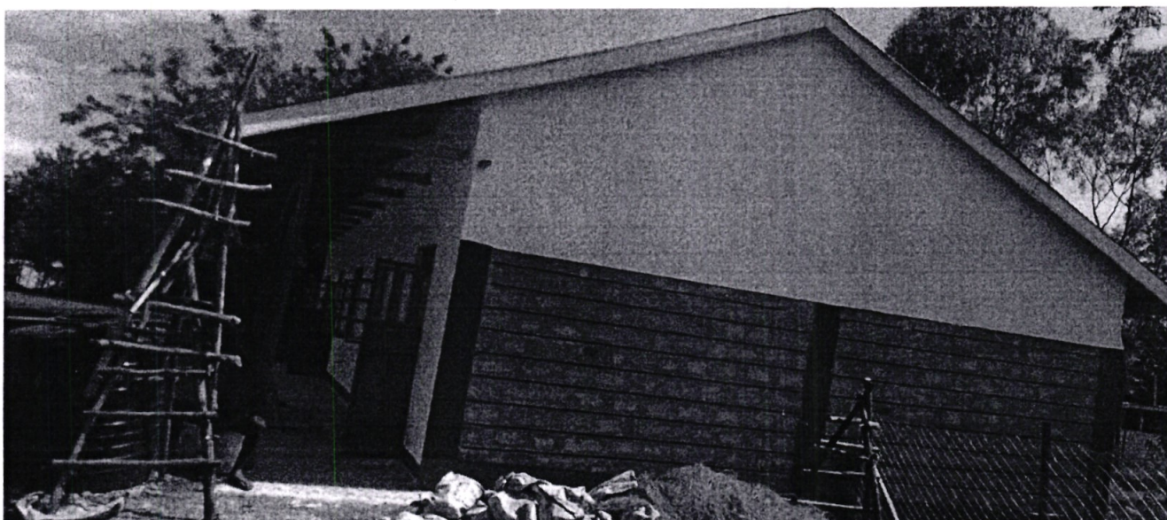
Onjiko Kobong'o Mixed Sec School, Construction of 45 capacity science laboratory.
