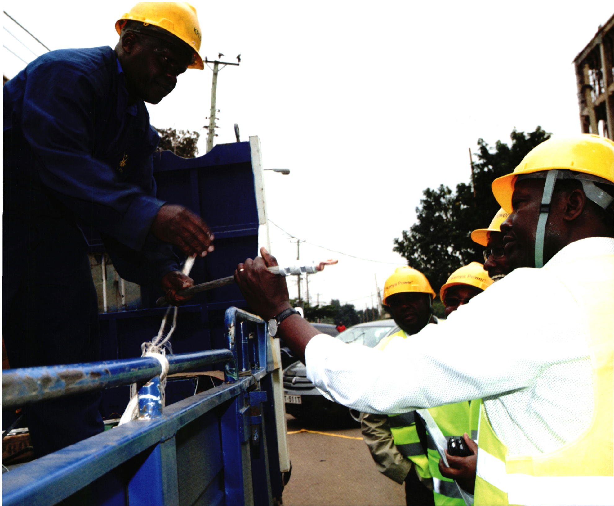
The Cabinet Secretary for Energy and Petroleum, Mr. Davis Chirchir, inspects an electric cable during a Boresha Umeme programme in Nairobi
