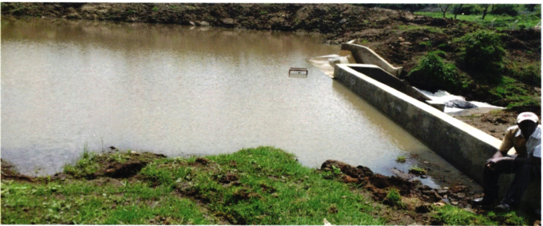
Figure 23: Nyaoroko Pan in Gilgil , Nakuru County where Land Waste is high but 60 acres of land have been reclaimed.
