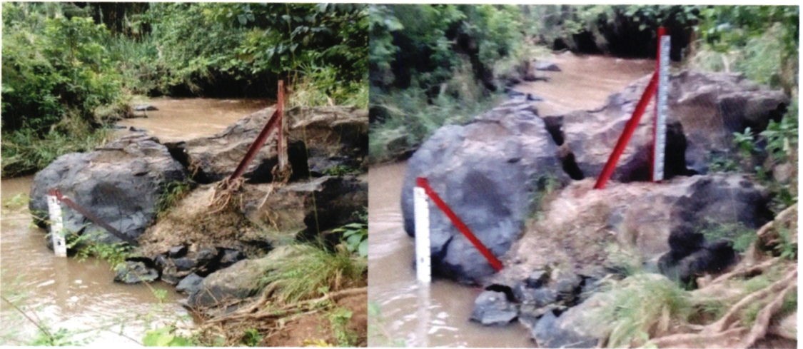
Figure 9: Rehabilitation at Awach Kajulu 1HA14 in Kisumu
