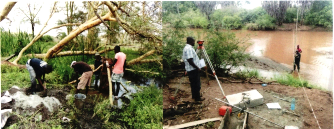
Figure 7: Installation of Tsavo RGS at Mombasa
