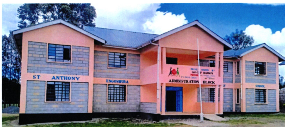
Figure 8: St. Anthony Engoshura Secondary School
