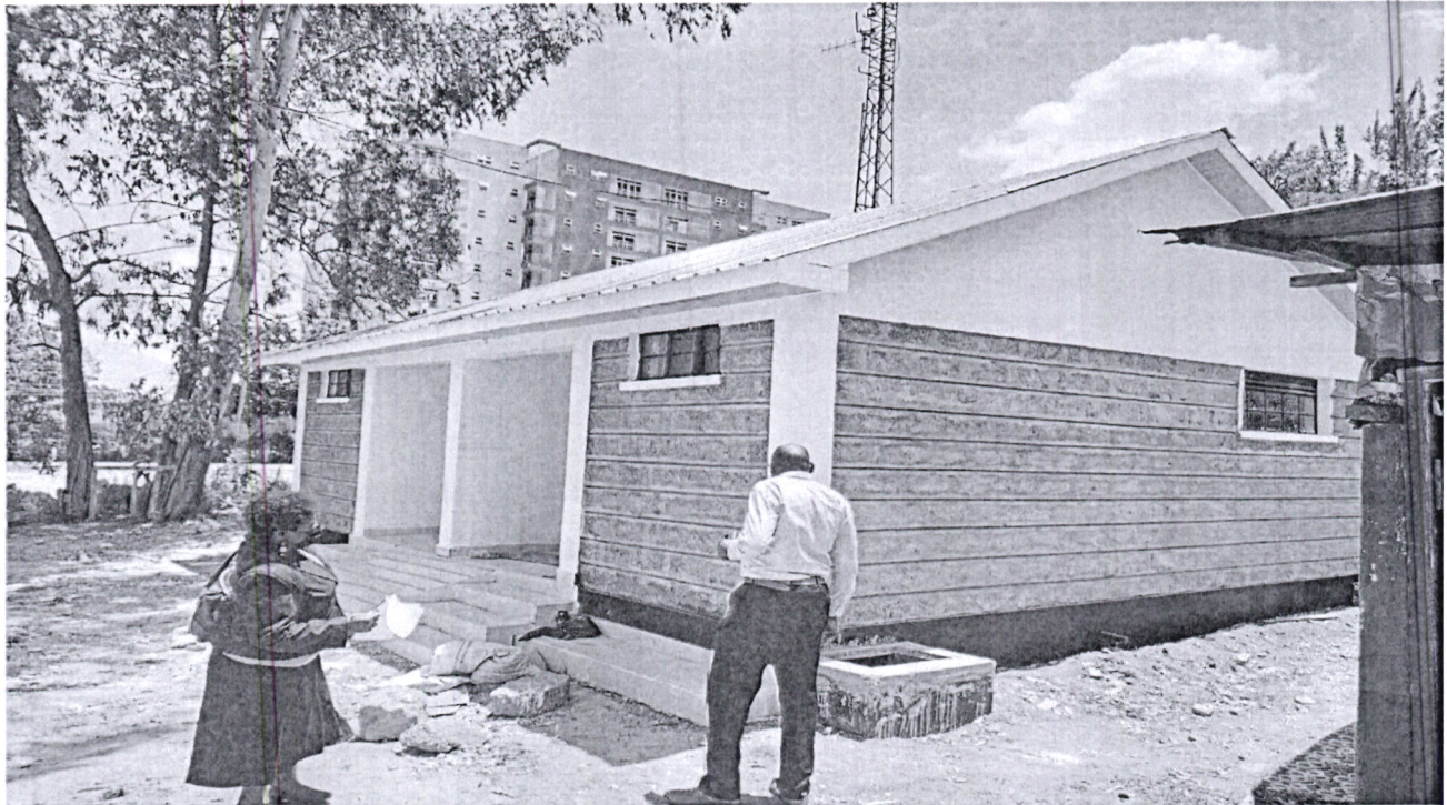
Figure 3: Construction of Toilet Block at Kilimani Police Station
