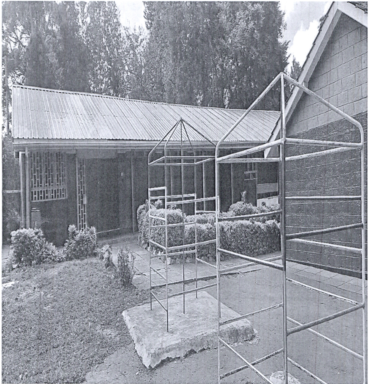
Figure 3: Renovation Works at Lavington Primary School
