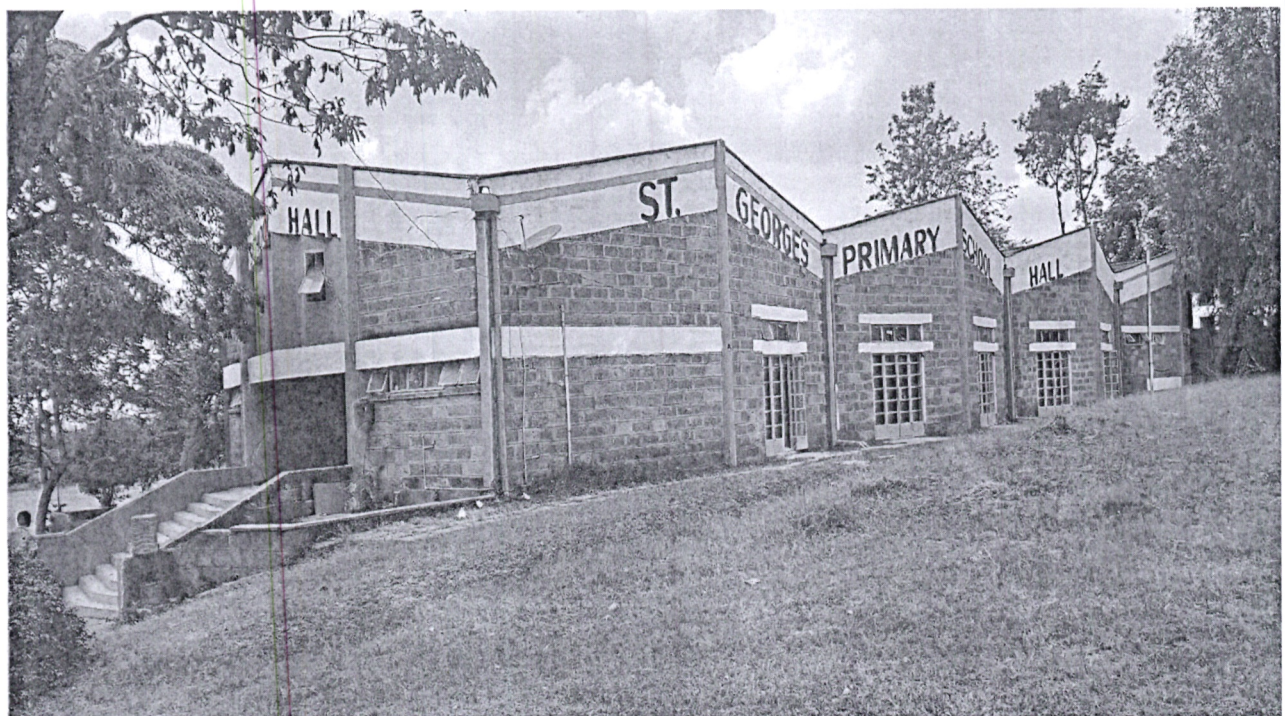
Figure 2: Renovation of Multipurpose hall at St. Georges Primary School
