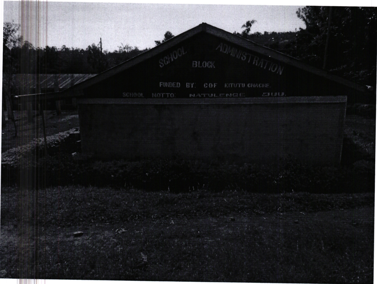
KITUTU CHACHE NORTH NG CDF PROJECT-ADMINISTRATION BLOCK CONSTRUCTED BY NG-CDF AT ERAMBA SECONDARY SCHOOL
