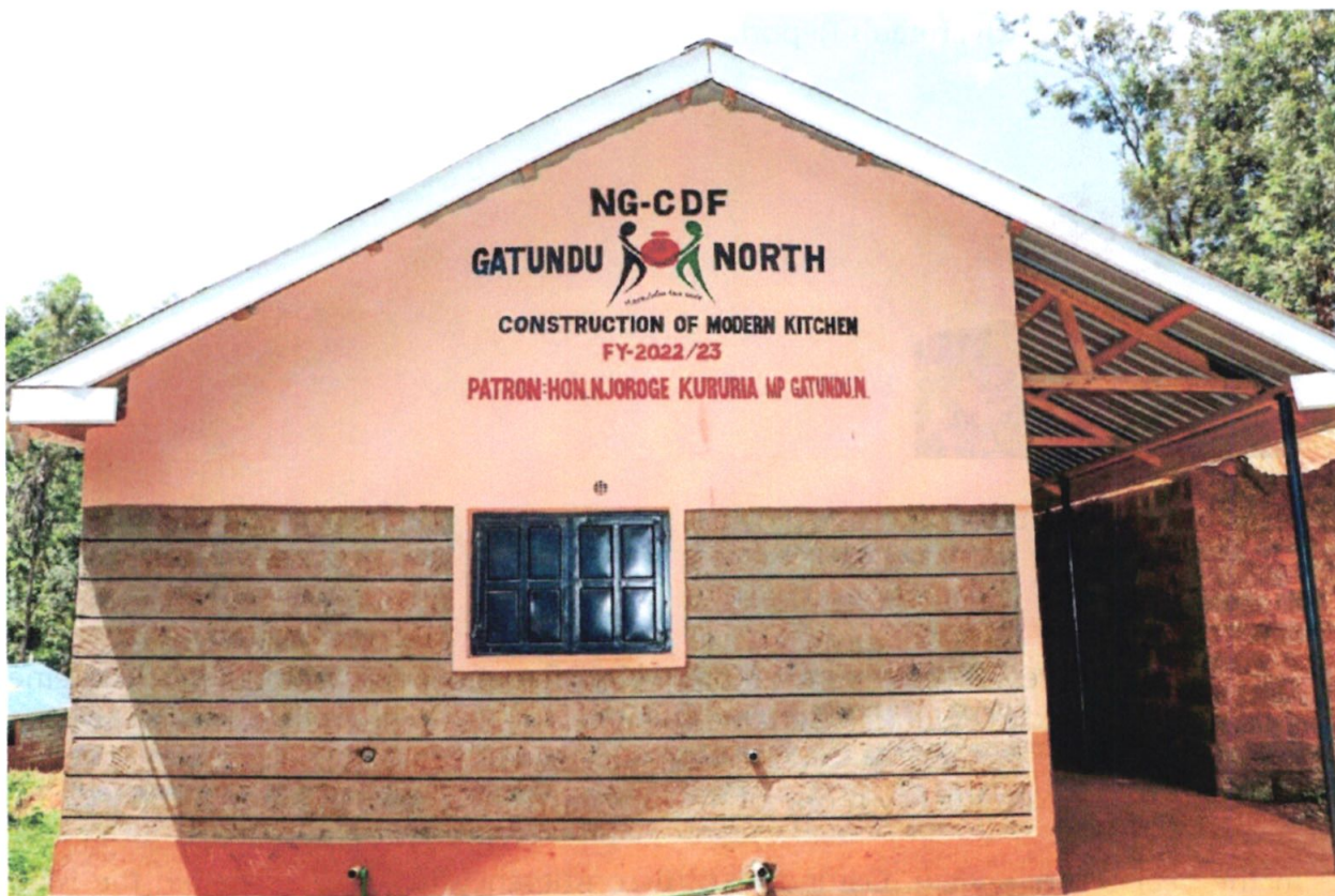
MWEA PRIMARY SCHOOL - KITCHEN
