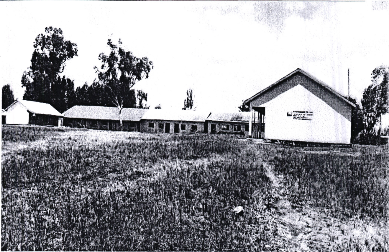
Nyamagogwi Secondary school Construction of two classrooms FY 202021
