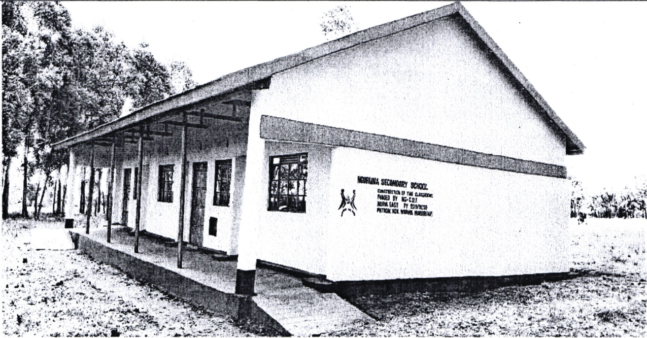
Nguruna Secondary School Construction of two classrooms FY 20202021
