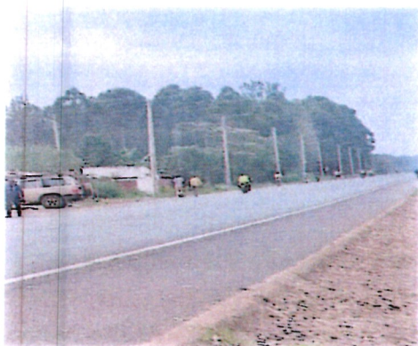
Street lights installed at Mosoch, Nyamira County
