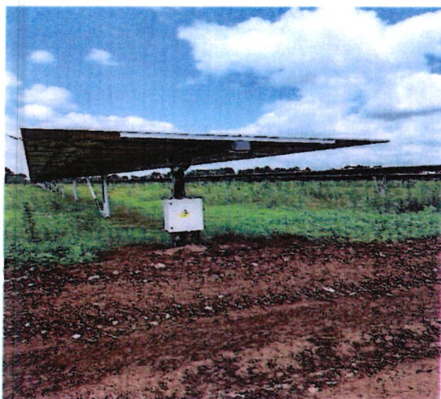
Installed solar panels at Alten Kesses 40MW solar power plant
