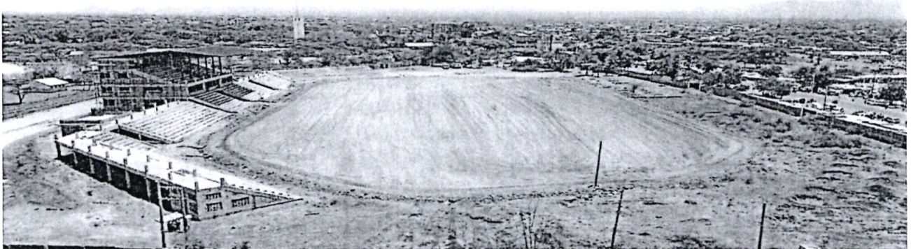
On-going construction of Isiolo Stadium
