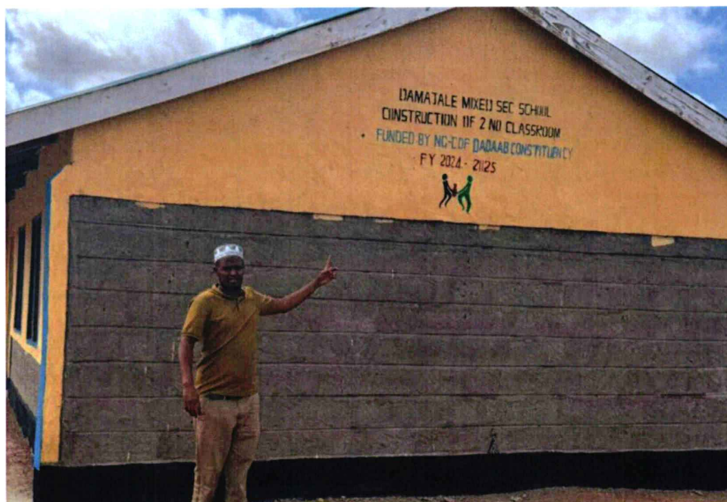
Construction of 2no classrooms at Damajaley Mixed Secondary School
