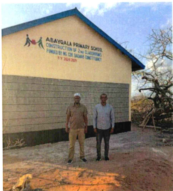
Construction of 2nd classrooms at Abaqaila Primary School
