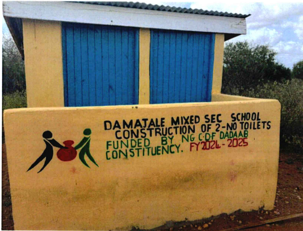
Construction of 2no toilets at Damajaley Mixed Secondary School
