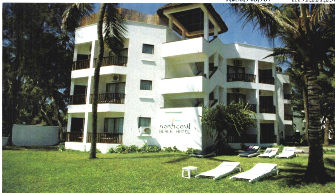
The refurbished North Coast Beach Hotel
