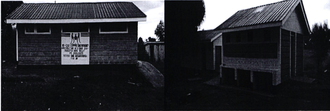
MAHINDU PRIMARY SCHOOL BIO DIGESTER
