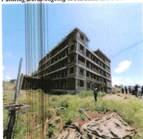
Ongoing Construction of Marsabit High court
