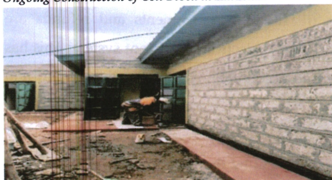
Painting works ongoing in Karatina cell block
