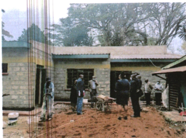
Ongoing Construction of Cell Block in Karatina
