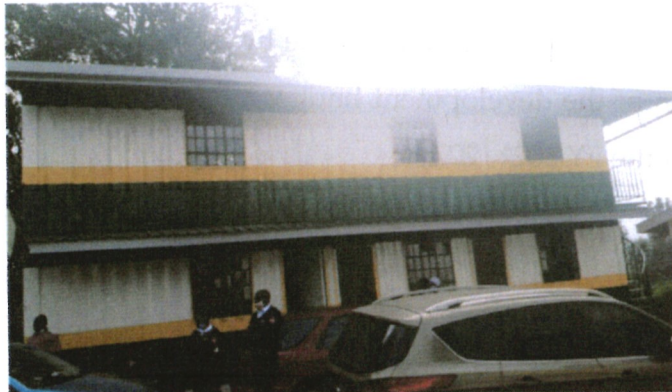
Prefabricated Container at Kandara Law Courts
