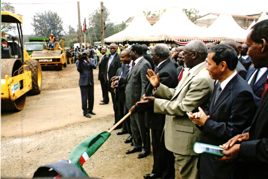
President Mwai Kibaki flags off construction of the Nairobi Western Ring Road in Nairobi on 12th August, 2011.
