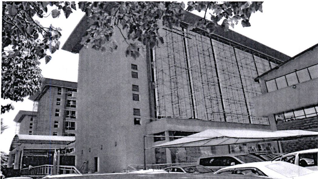
The New Mitihani House (Ongoing Project)
