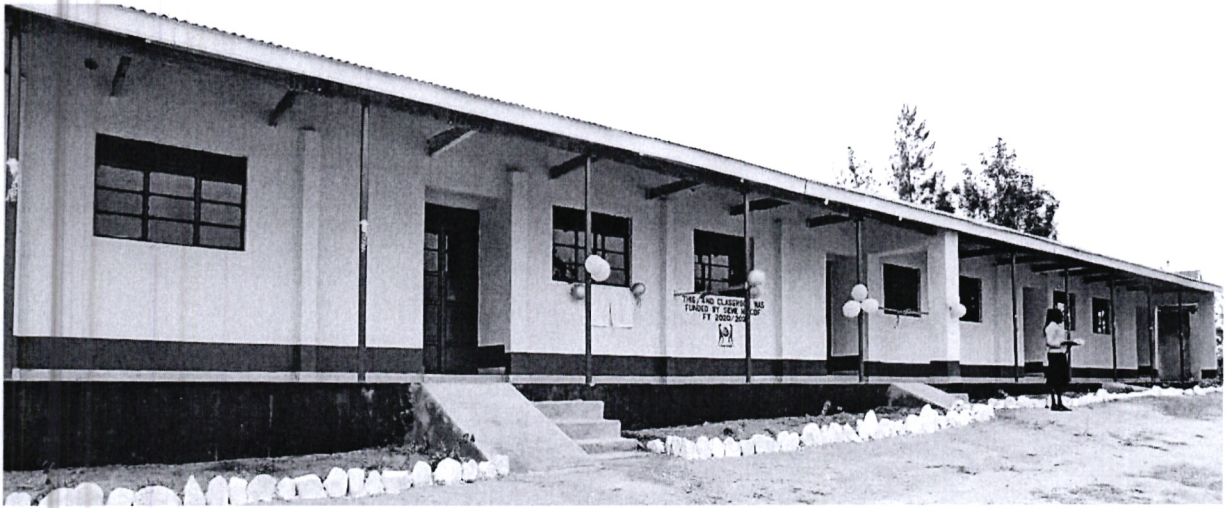
Fig 6: Omore Primary School – Classroom Construction
