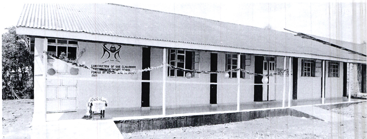
Fig 5: Akonya Primary School – Classroom Construction
