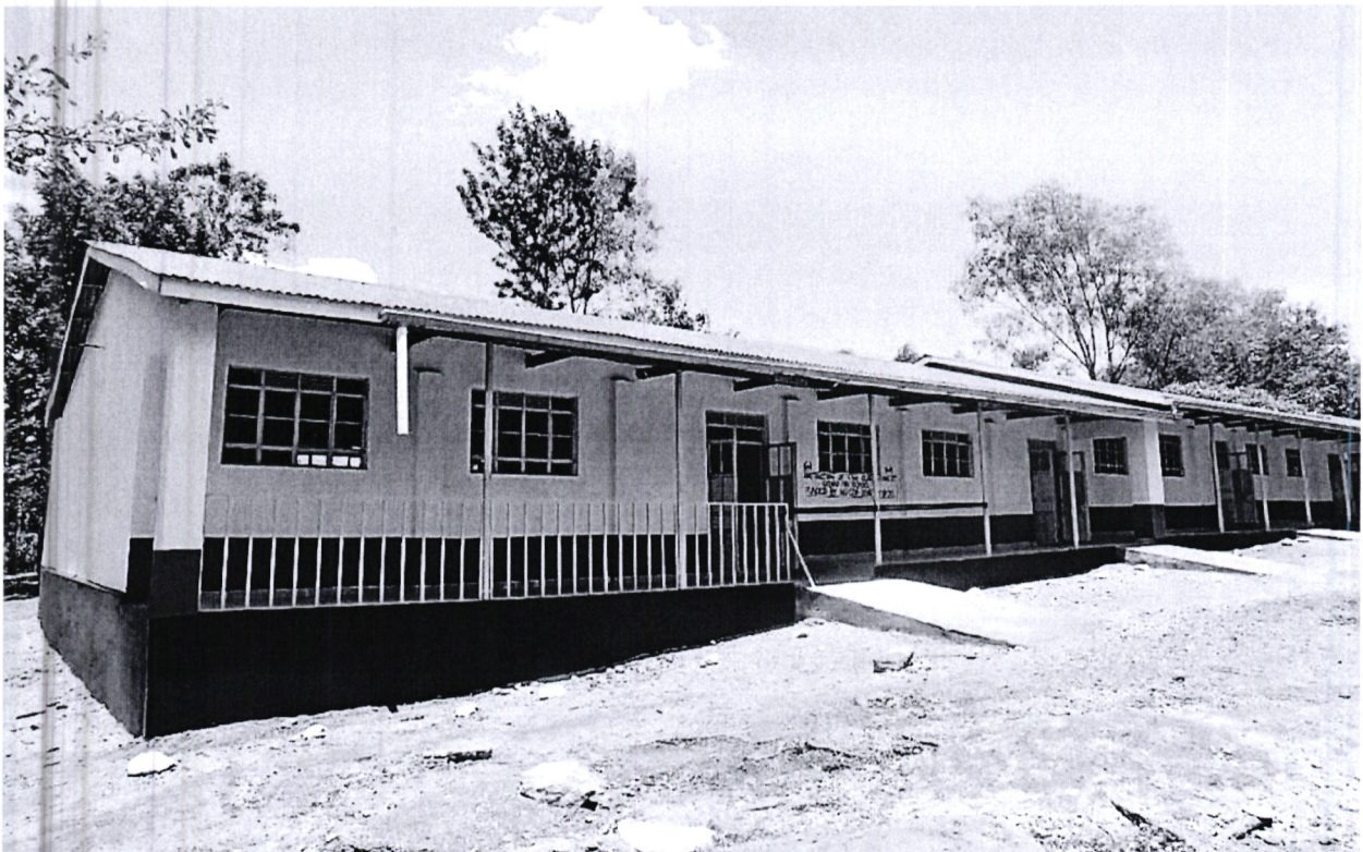
Fig 3: Diemo Primary School – Construction of 4 Classrooms
