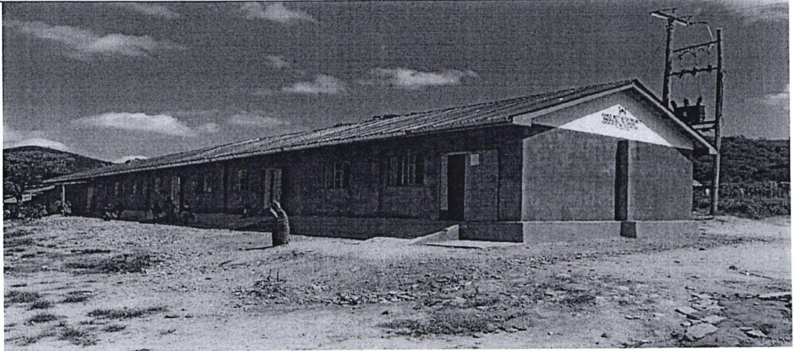
Kwakaleli Primary school-5NO.classrooms renovated, funds approved in FY 2018/2019
