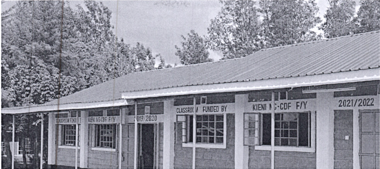
MWIYOGO PRIMARY SCHOOL CLASSROOM CONSTRUCTION
