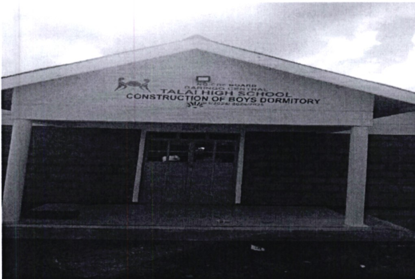
Talai High School-construction of boys dormitory
