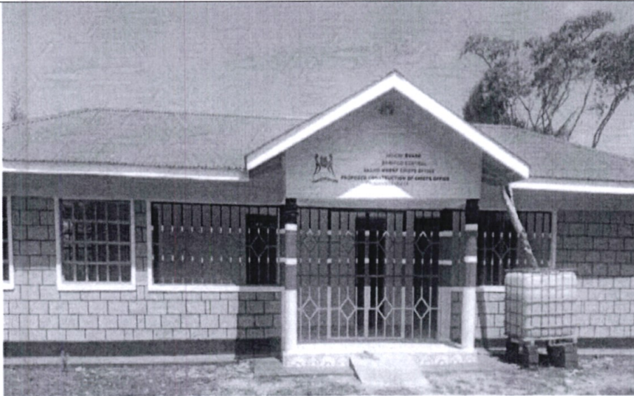
Sacho Mosop chiefs office -construction of chiefs office
