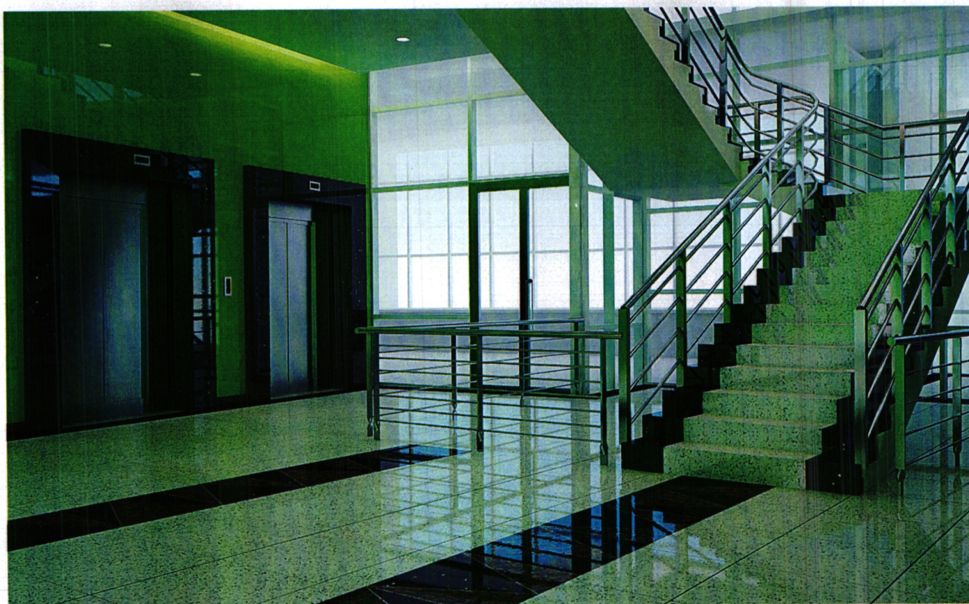
A Section of Konza complex under construction and Exterior finishes.
