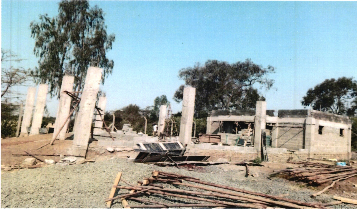
Figure 1: Ongoing Construction of Student Cafeteria funded by the BOG
