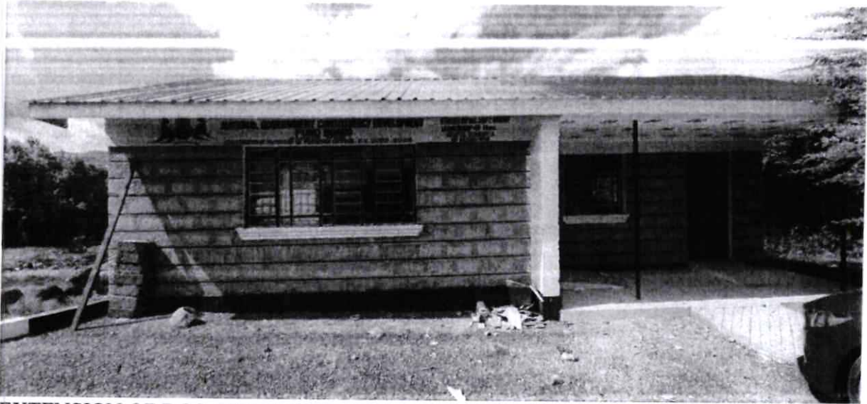
EXTENSION OF DCC OFFICES BLOCK
