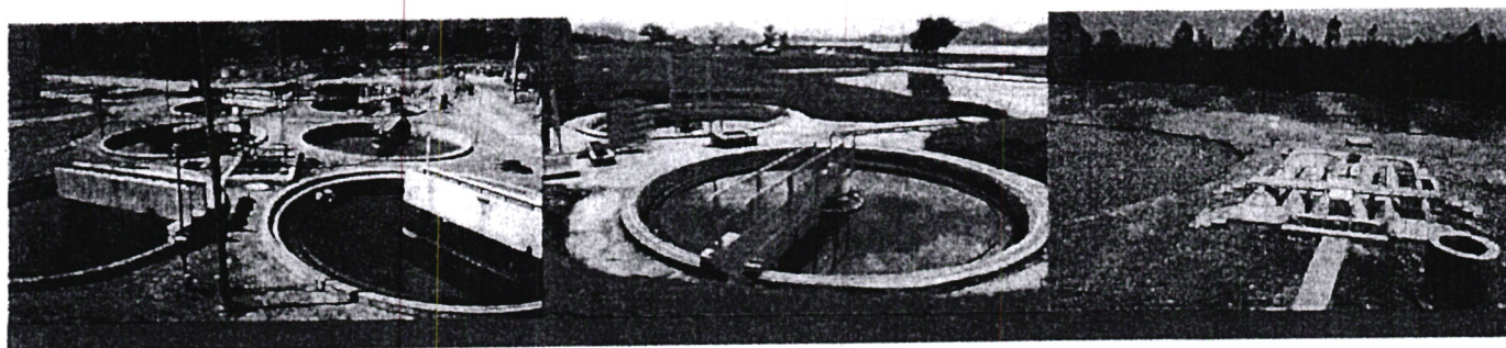
Picture 10: The Completed rehabilitation of Kisumu (1), Homa Bay (2) and Bomet(3) Sewerage treatments facilities in Kenya
