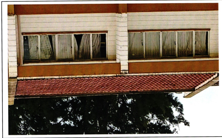
Figure 17: Repaired Hostel Roof
