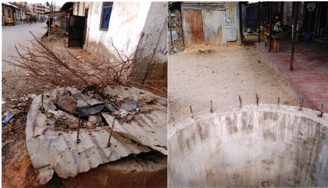
Figure 11: Manholes Constructed Alongside Informal Business Structures
