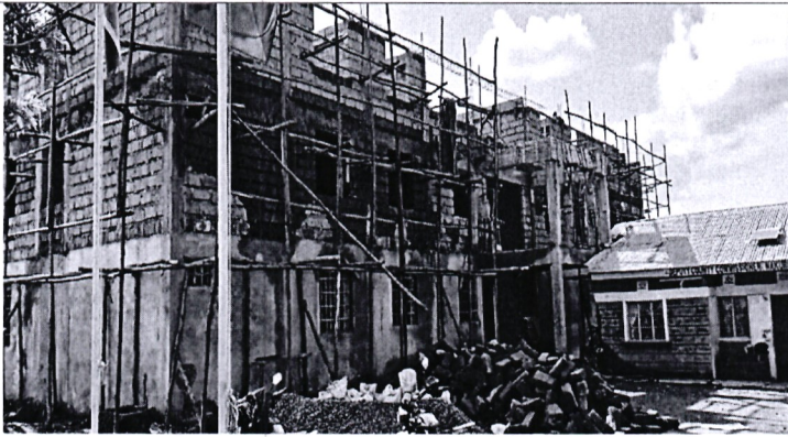
ON-GOING CONSTRUCTION OF D.C.C HEAQUARTERS OFFICES AT KAPKURES
