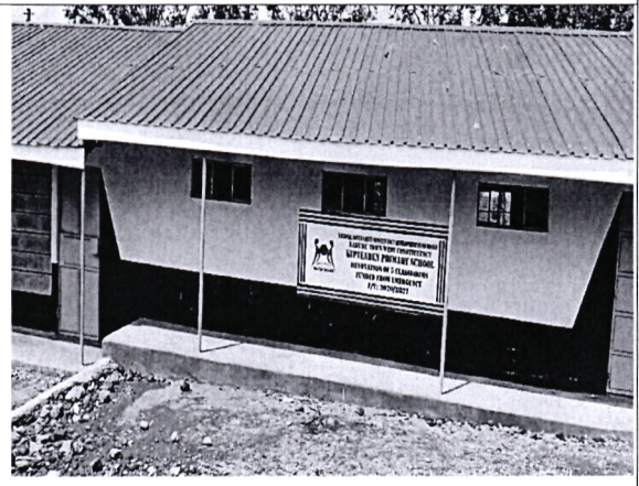
COMPLETE- RENOVATION OF 5 CLASSROOMS AT KIPTENDEN PRIMARY SCHOOL
