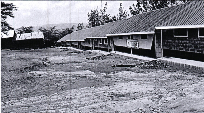
COMPLETE- REHABILITATION OF 5 CLASSROOMS AT KIPTENDEN PRIMARY
