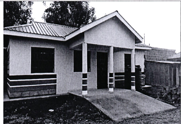
ON-GOING CONSTRUCTION OF PARKVIEW CHIEF/ASSISTANT CHIEF OFFICE
